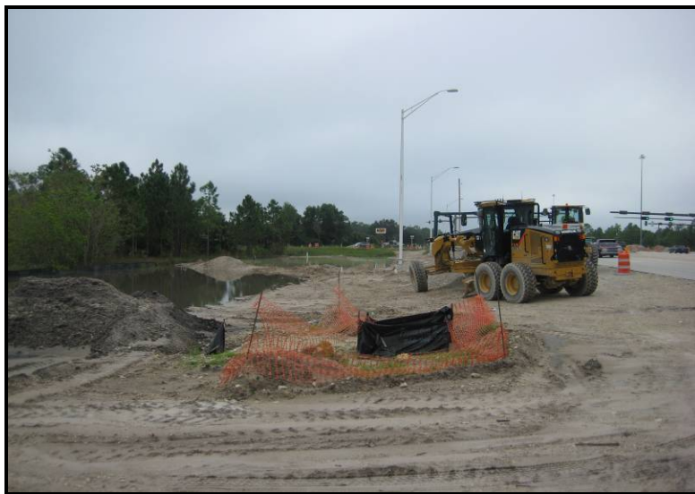
Photo 1. Current conditions of the southeast interchange area.
