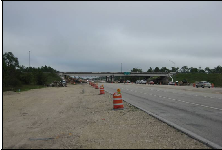
Photo 2. Looking north at the CR 951/I-75 Interchange.
